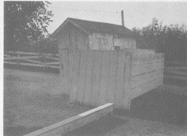
Unsanitary and out-dated toilet facilities.
