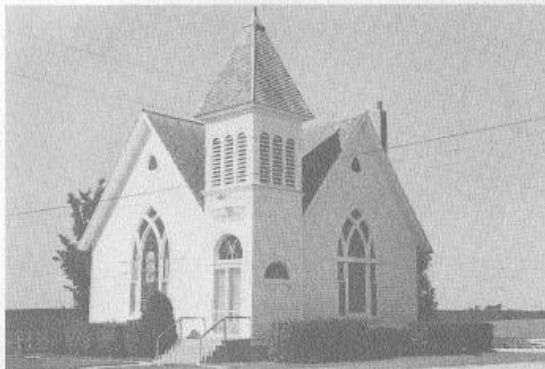
Present building completed.
